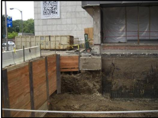
*Figure 8: View of Timber Shoring System*
